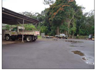
A vehicle storage shed is used to store vehicles and landscape equipment.
