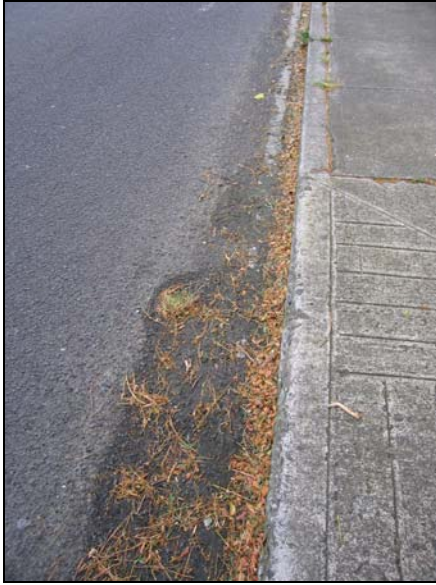
Debris accumulated along roadway curb and storm drain inlet
