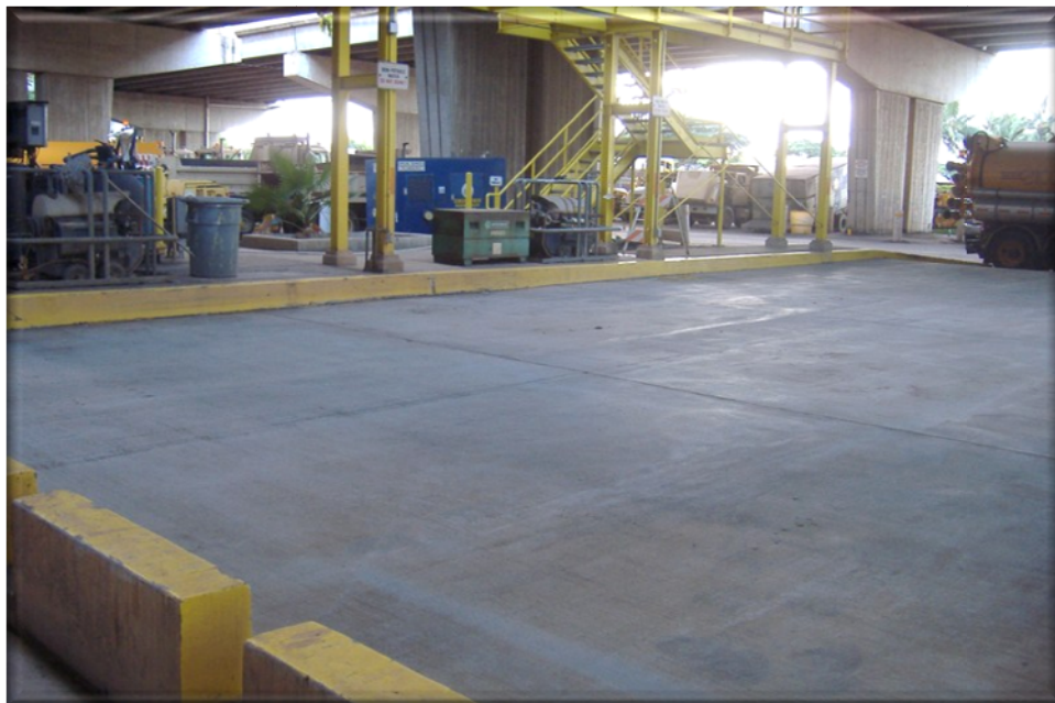
Keehi Baseyard vehicle and equipment wash rack is designed to contain, collect, treat, and recycle wash water for vehicle washing.
