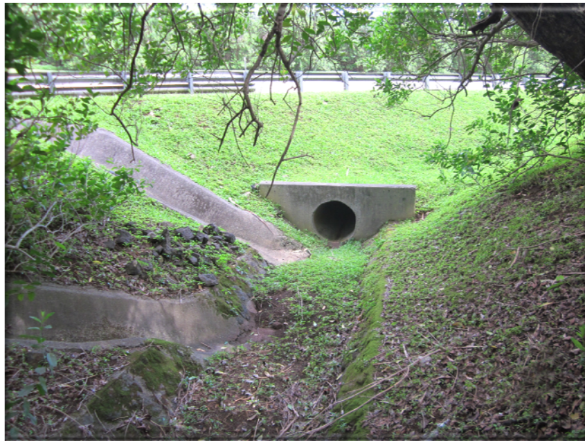
Inspectors document an existing connection to the MS4.
