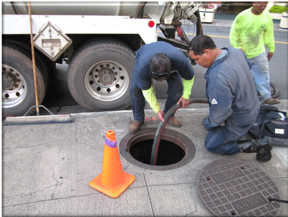
Industrial vacuum trucks are utilized to clean the storm drains.
