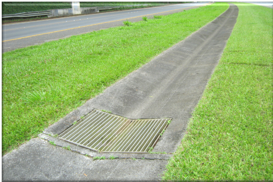
Vegetated buffers trap sediment and reduce storm water runoff by providing opportunities for storm water infiltration.
