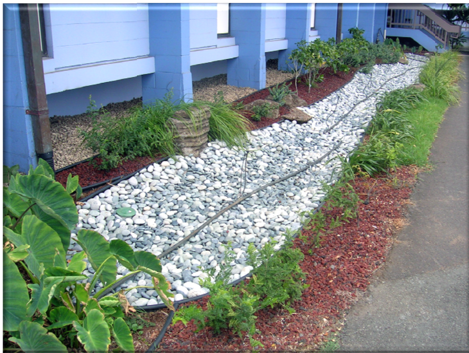
The Kakoi Rain Garden at the DOT-HWYS office is a Low Impact Development Best Management Practice.
