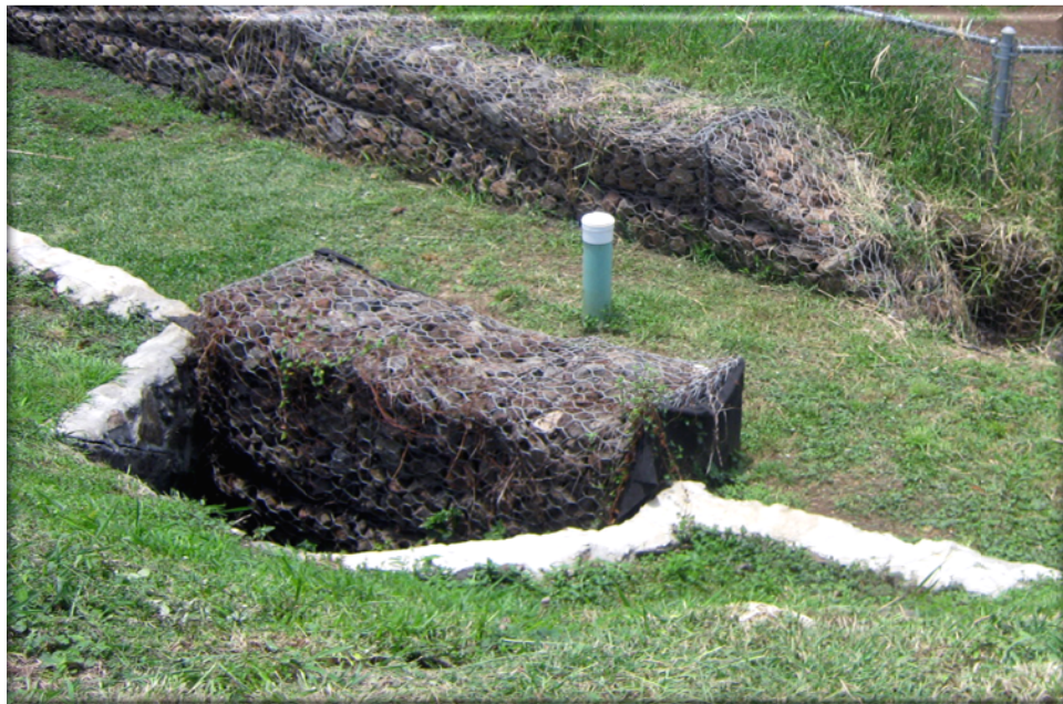
Constructed bioswales provide a location for storm water to collect and infiltrate through an engineered soil matrix before entering an under drain system that connects to the MS4.
