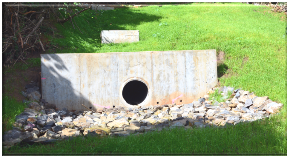
This previously eroded outfall was completely repaired and reconstructed. A rip rap apron provides protection from future erosion.
