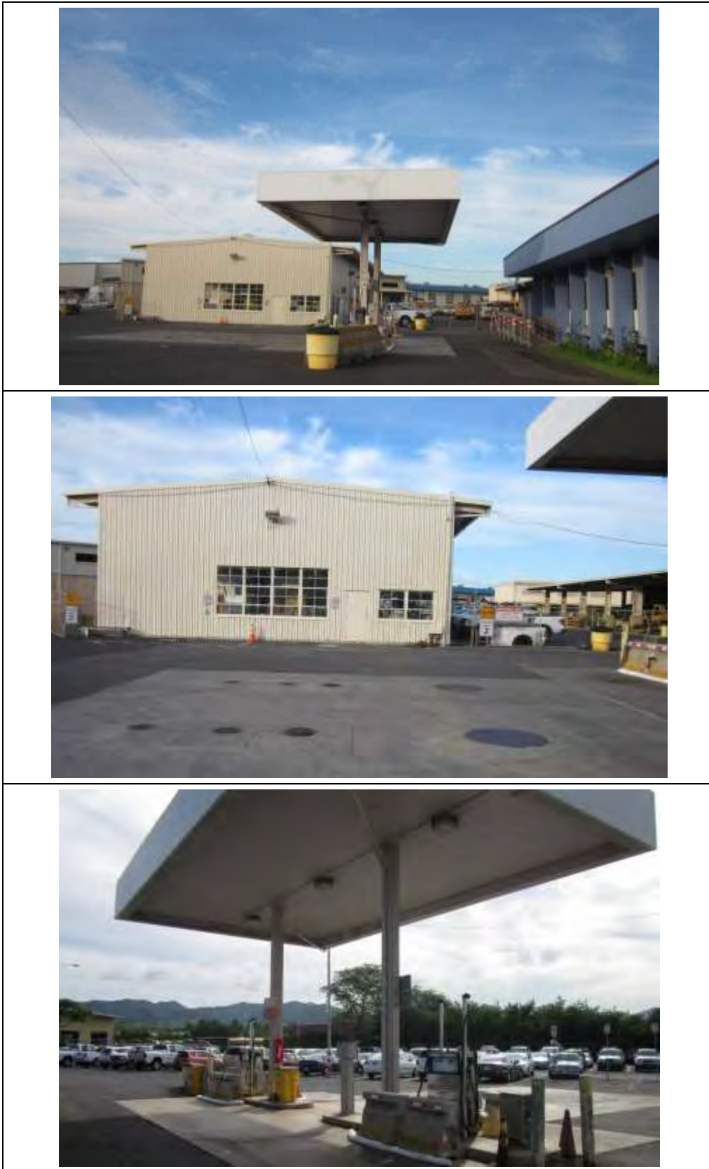
FIGURE 3-4: BASEYARD FUNCTIONAL AREAS – FUEL STATION AND USTs
