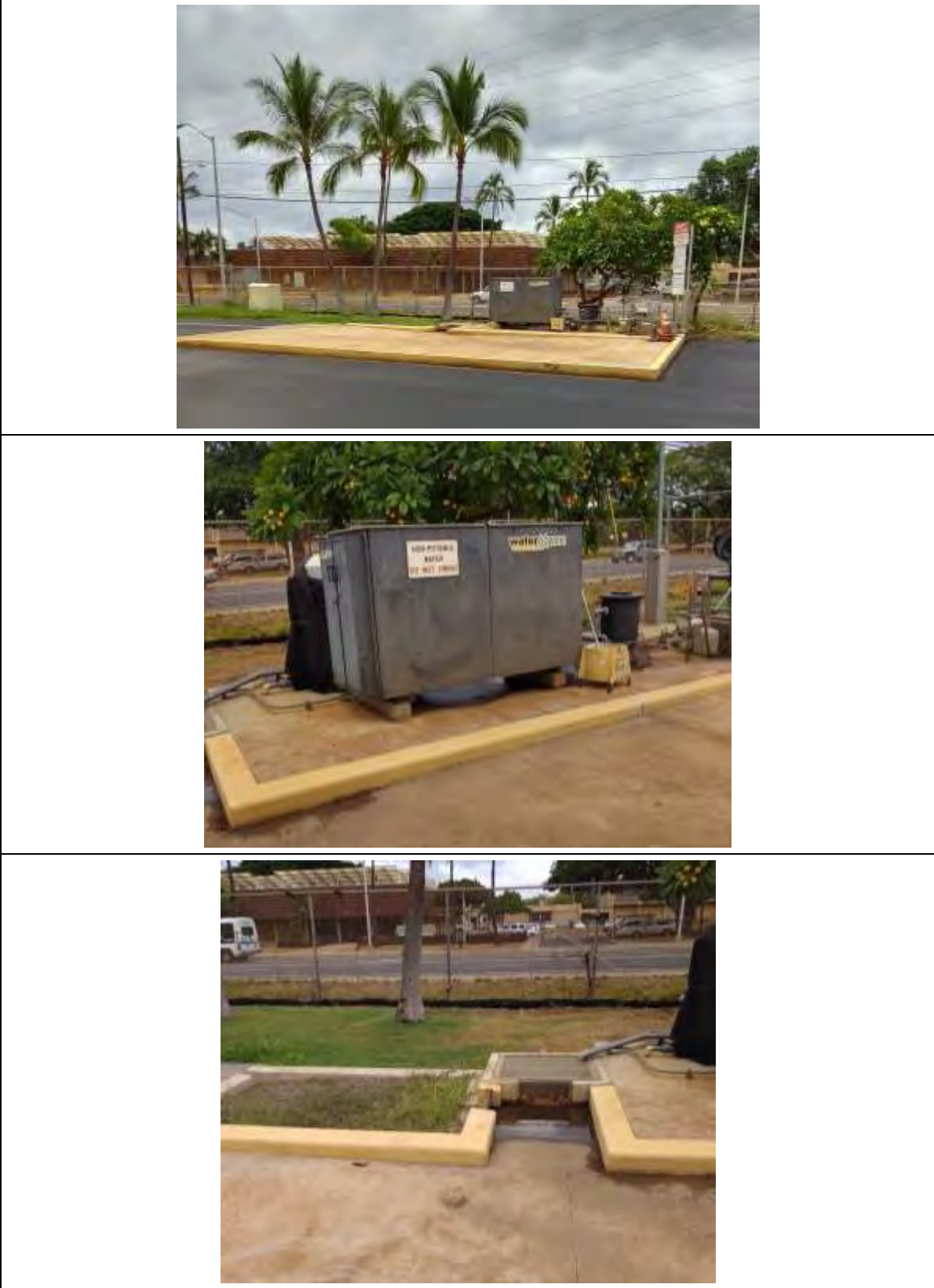
FIGURE 3-3: BASEYARD FUNCTIONAL AREAS – VEHICLE AND EQUIPMENT WASH RACK
