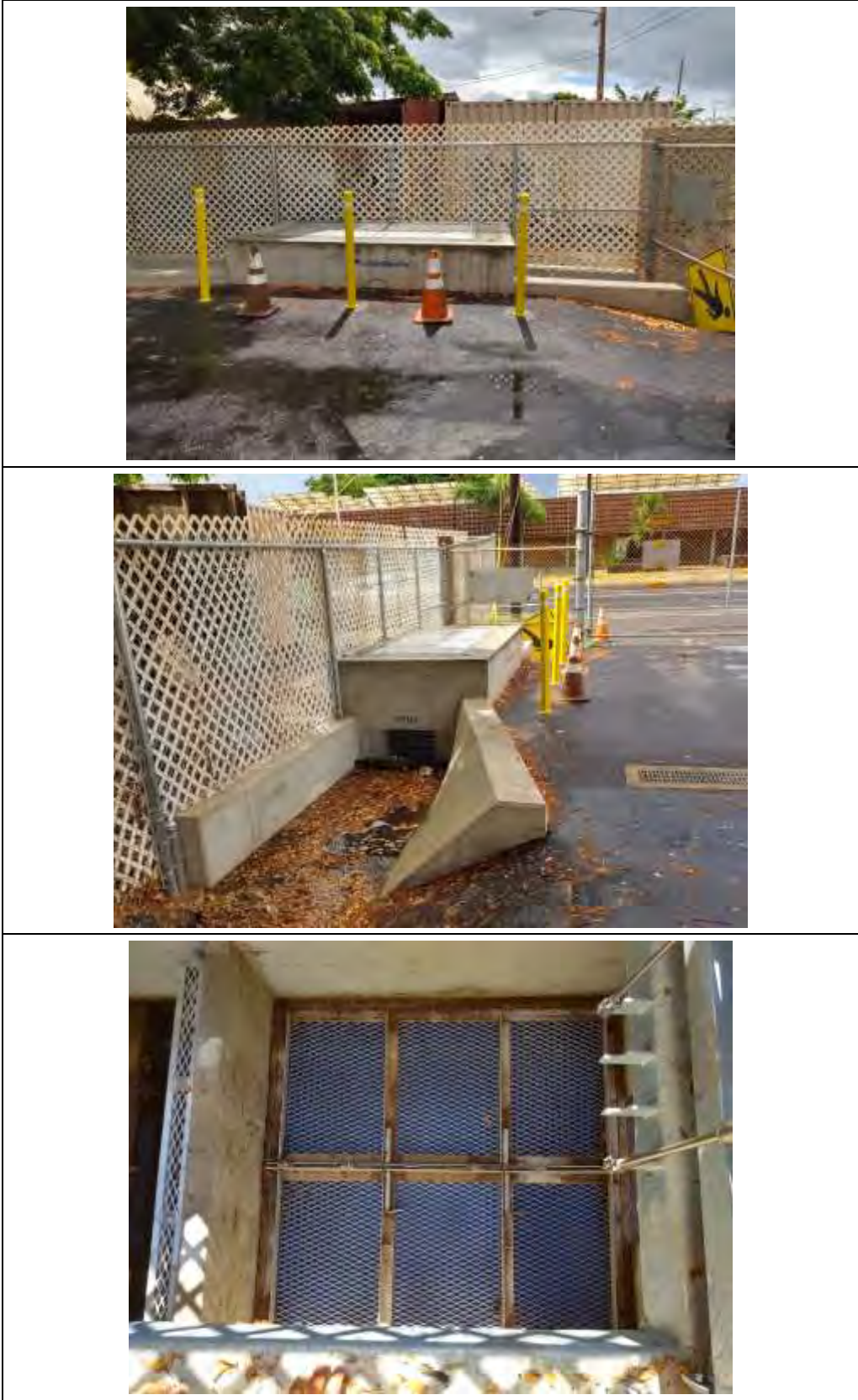
FIGURE 3-9: BASEYARD FUNCTIONAL AREAS – WATER POLISHER
