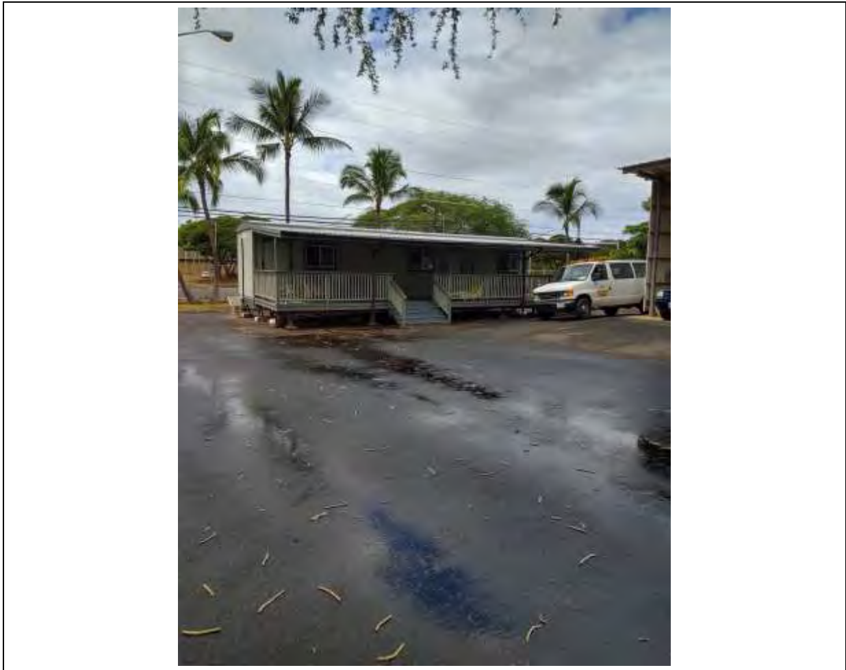
FIGURE 3-1: BASEYARD FUNCTIONAL AREAS – ADMINISTRATIVE BUILDING
