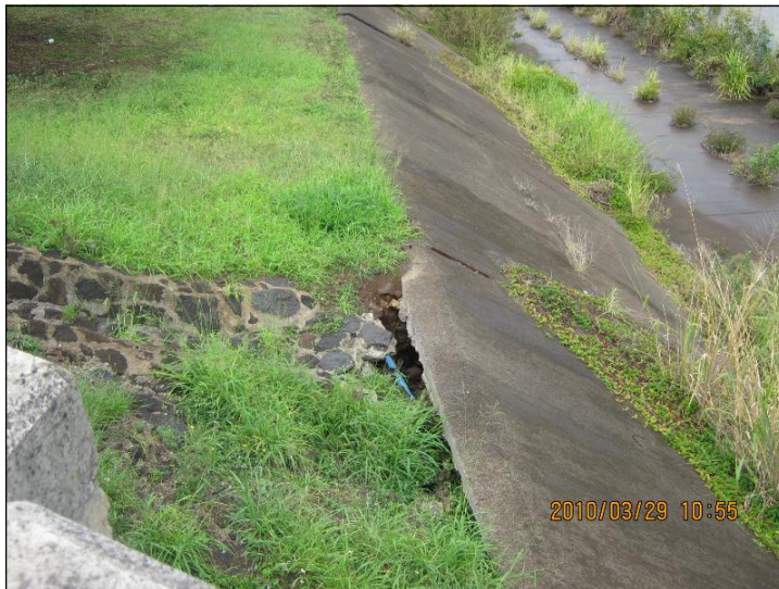
Photo 1: CRM spillway to concrete lined channel
