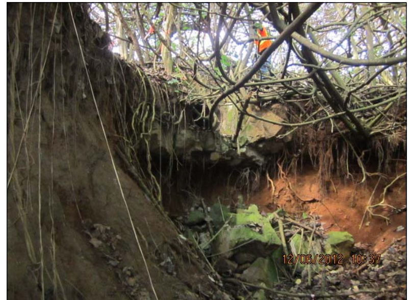
Photo 2: Outfall erosion
