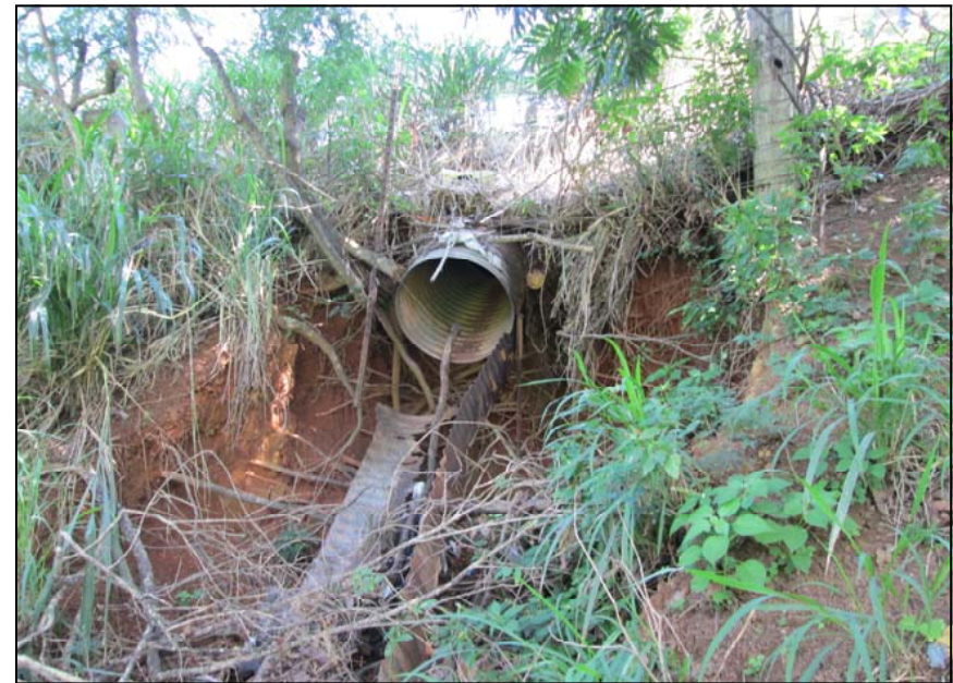
Photo 2: Outfall erosion
