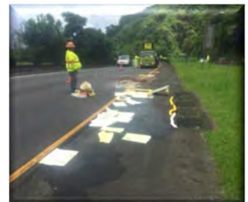
Use absorbent material.
