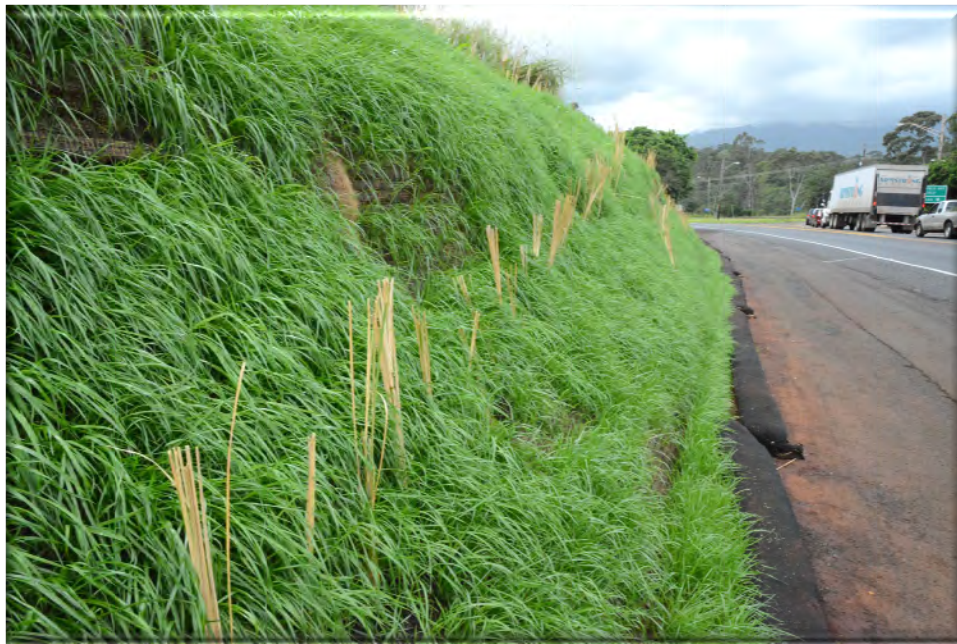
Repair of this eroded slope involved applying a mixture of grass seed, fertilizer, and mulch, which was then secured in place using erosion control fabric. The newly planted grass has grown significantly, and completely obscures the erosion control fabric from view.
