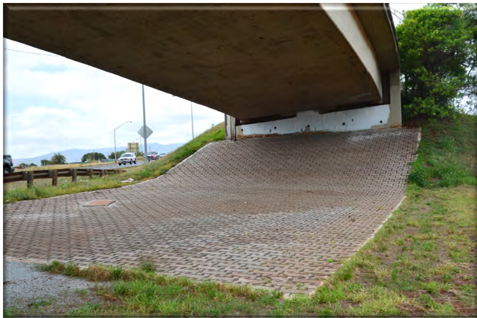
Articulated Concrete Block Mat Systems are an effective, economic method of erosion control in areas where establishing new vegetation is difficult.
