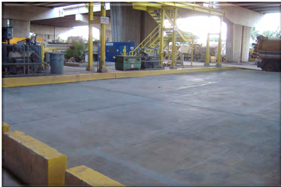
Keahi Baseyard vehicle and equipment wash rack is designed to contain, collect, treat, and recycle wash water for vehicle washing.
