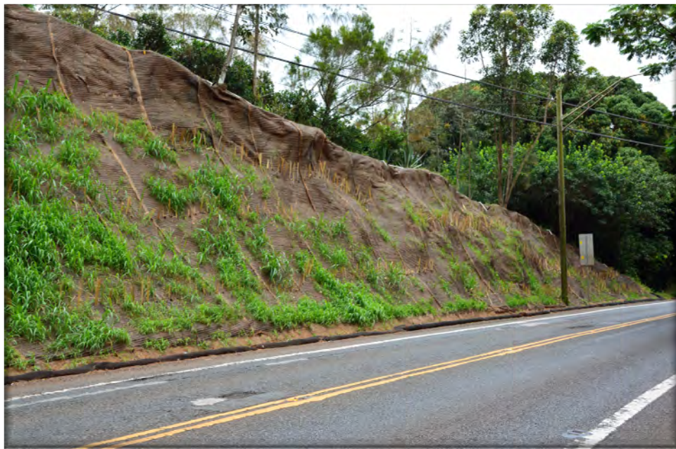
This eroded slope was repaired by applying a mixture of grass seed, fertilizer, and mulch, which was then secured in place using erosion control fabric. The newly planted grass is just beginning to sprout through the fabric.
