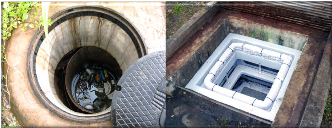
Hydrodynamic separators (left) and storm catch basin filter systems (right) trap trash, debris, and sediment before it can enter the MS4 and be discharged to the ocean.
