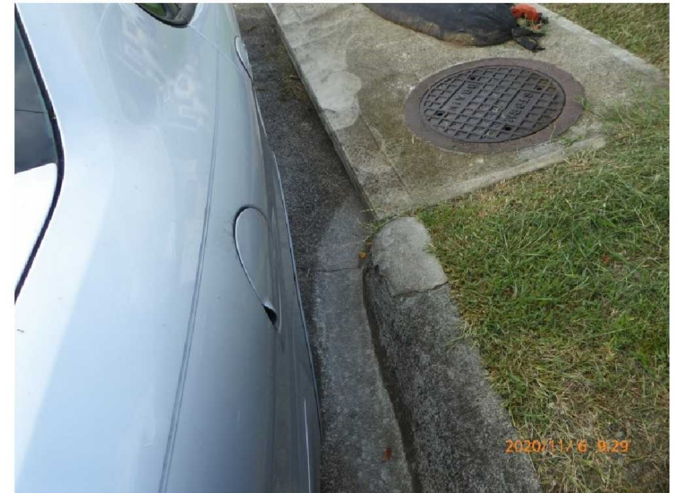
Concrete slurry appears to have entered an unprotected catch basin.
