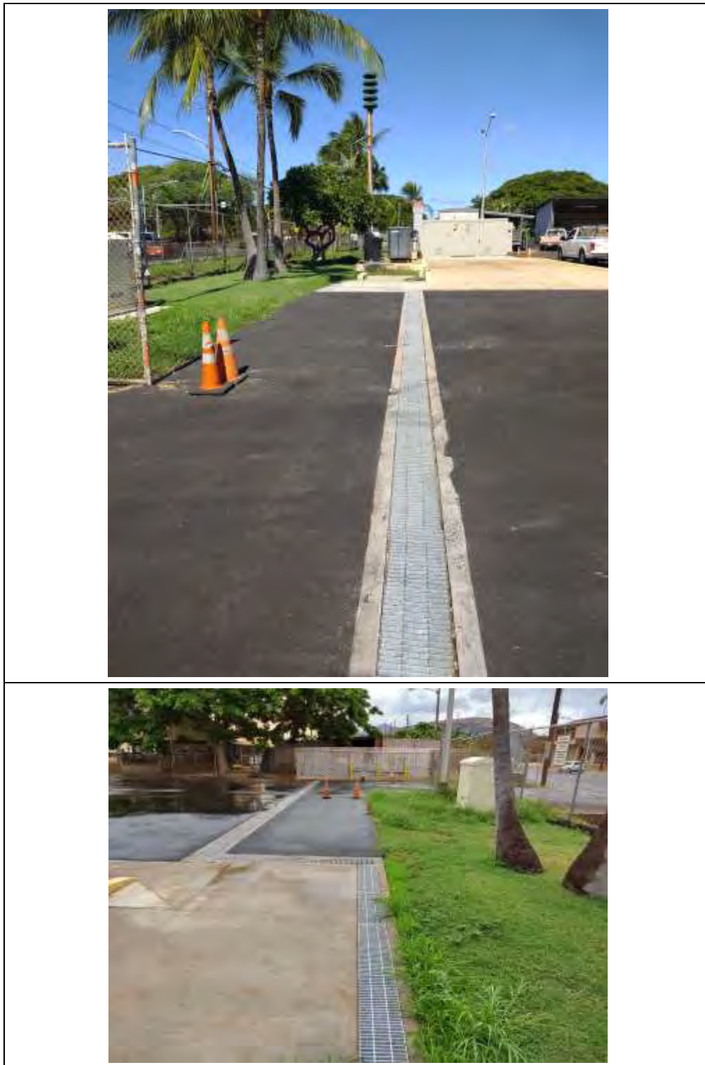
FIGURE 3-8: BASEYARD FUNCTIONAL AREAS – TRENCH DRAIN
