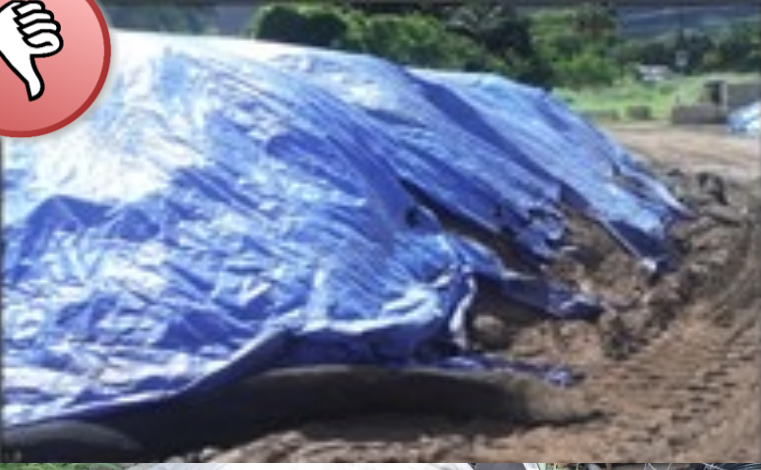
Torn cover/Gap in perimeter
