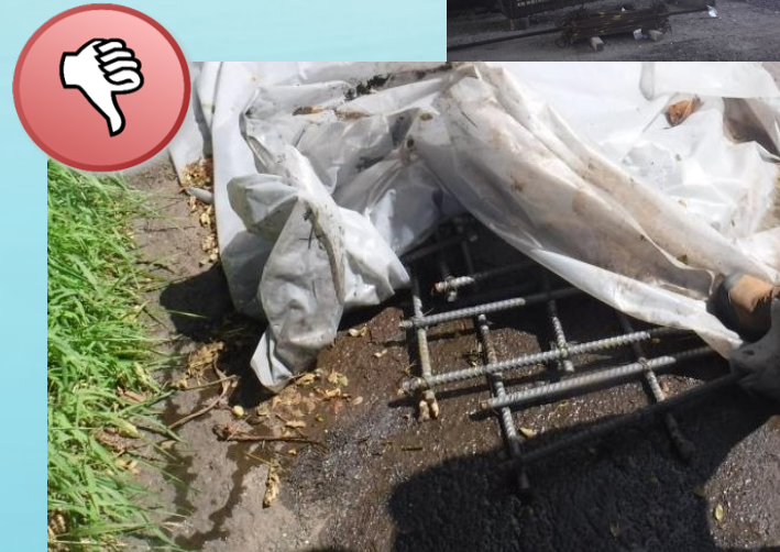
Covered not racked – laying in water
