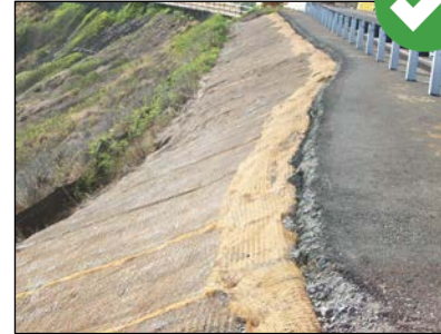
Check with manufacturer's specifications for erosion control matting anchorage requirements.
