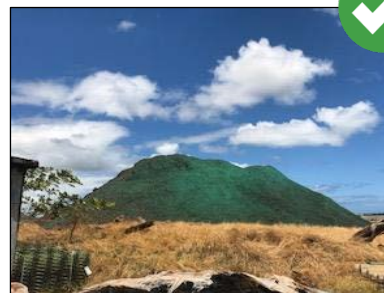
Soil binders can be used on large stockpiles to prevent erosion from wind and rain.
