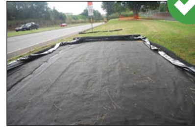
Store vehicles and equipment on a layer of geotextile filter fabric on top of 10 mil plastic sheeting when not being used.
