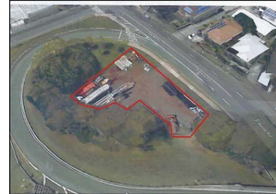
Aerial view of a construction staging area.
