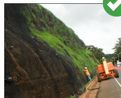
Phase disturbances and use stabilization techniques designed for steep grades if disturbance of steep slopes is unavoidable.
