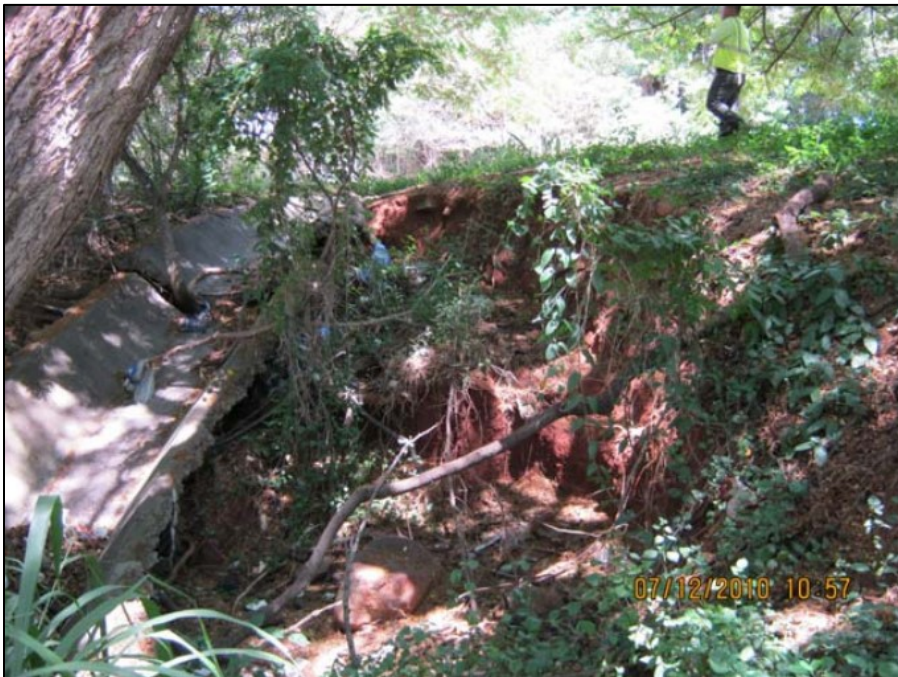
Erosion at outfall
