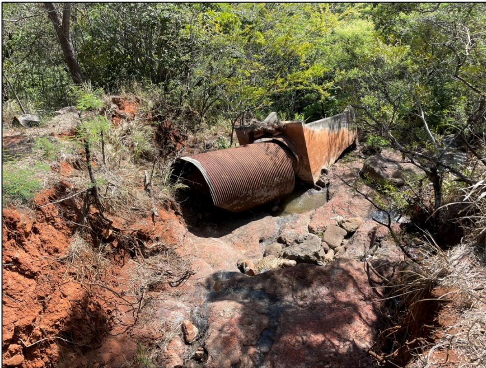
Failed concrete outlet structure downstream of outfall
