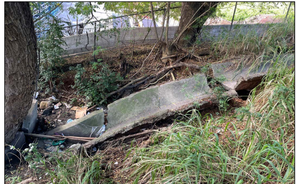
Failing concrete liner at outfall
