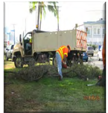
Remove and dispose of debris.
