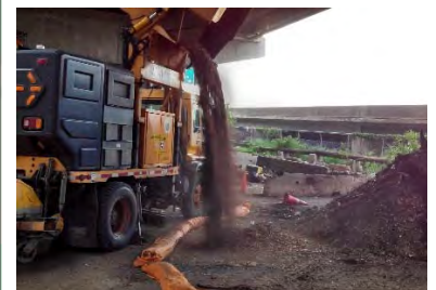
Use berms for stockpiling.
