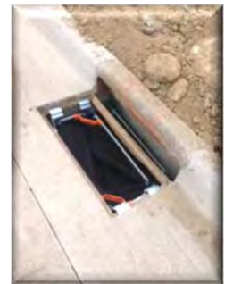
Protect stormwater drainage.
