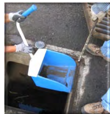
Clean storm drain.
