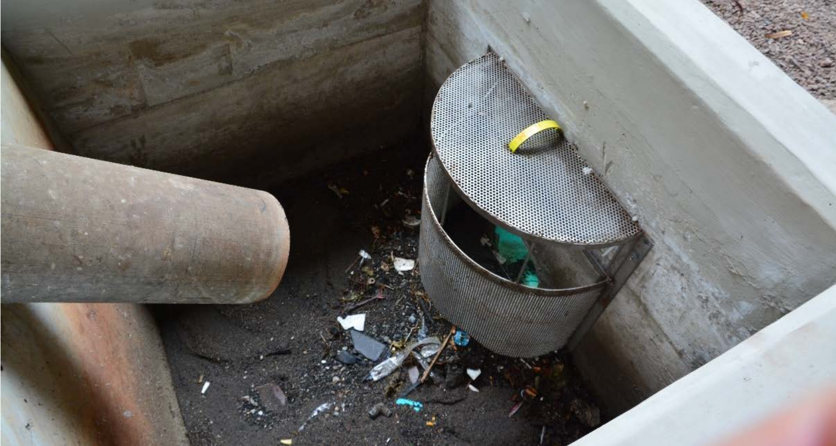
A downspout filter box captures pollutants under the H-1 Viaduct in the Waimalu Watershed.
