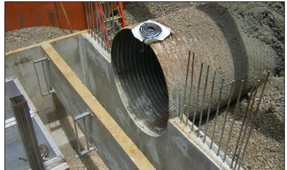
**Nutrient Separating Baffle Box during construction**
