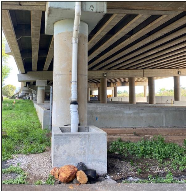
**Newly Constructed Downspout Filter Box**
