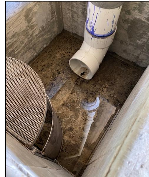
**Newly Constructed Downspout Filter Box**
