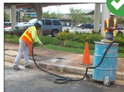
Properly vacuuming saw cut and boring slurry prevents the slurry from entering storm drain systems and adjacent waterbodies.
