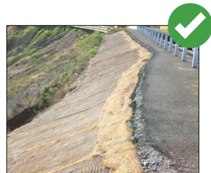
Check with manufacturer’s specifications for erosion control matting anchorage requirements.
