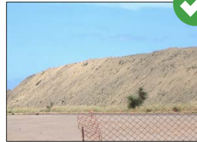
Use a tackifier, netting, or mechanical “punching” method to anchor mulch. Method depends on slope steepness, accessibility, soil conditions, and longevity.
