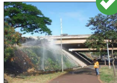
Temporary irrigation may be required for initial establishment of vegetation and sustained growth.
