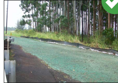
Mulches must be applied at the manufacturer's recommended rate to ensure uniform and effective coverage.
