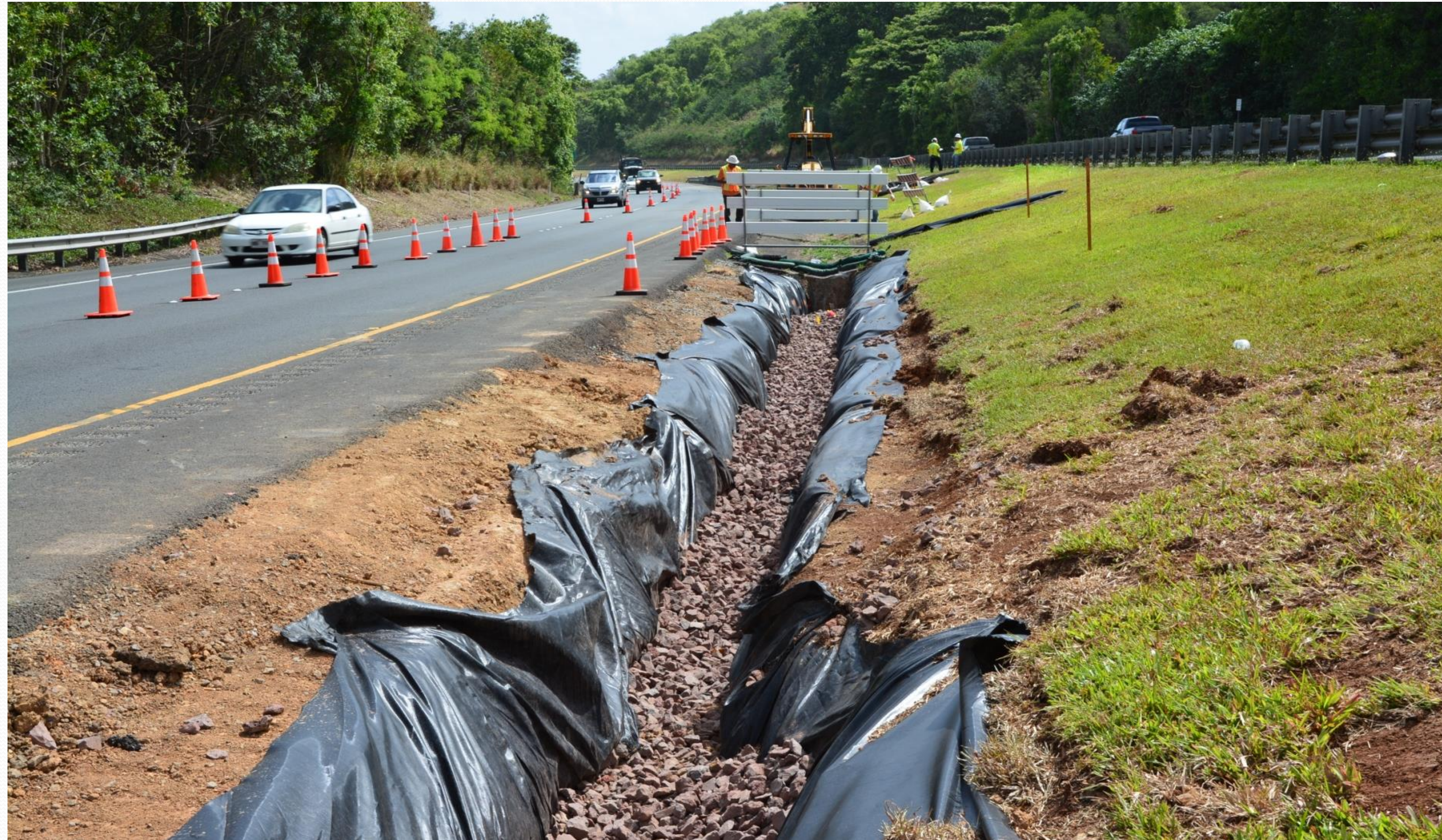
Enhanced/Bioswale Construction
