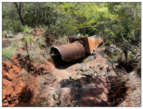
Failed concrete outlet structure downstream of outfall
