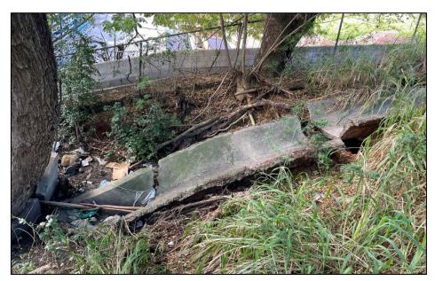
Failing concrete liner at outfall
