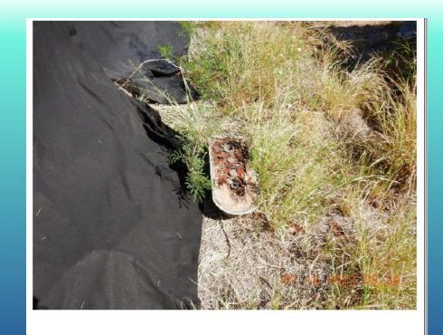
**Photo 2 Description:** Move materials stored beyond installed perimeter sediment control measures to within the staging area limits.
