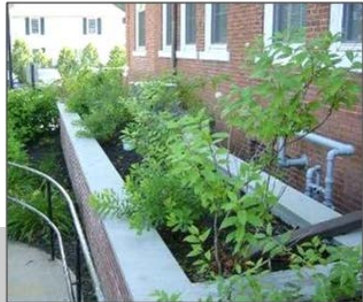
Infiltrating planter box designed to capture and treat rooftop runoff (Plymouth, MA).
