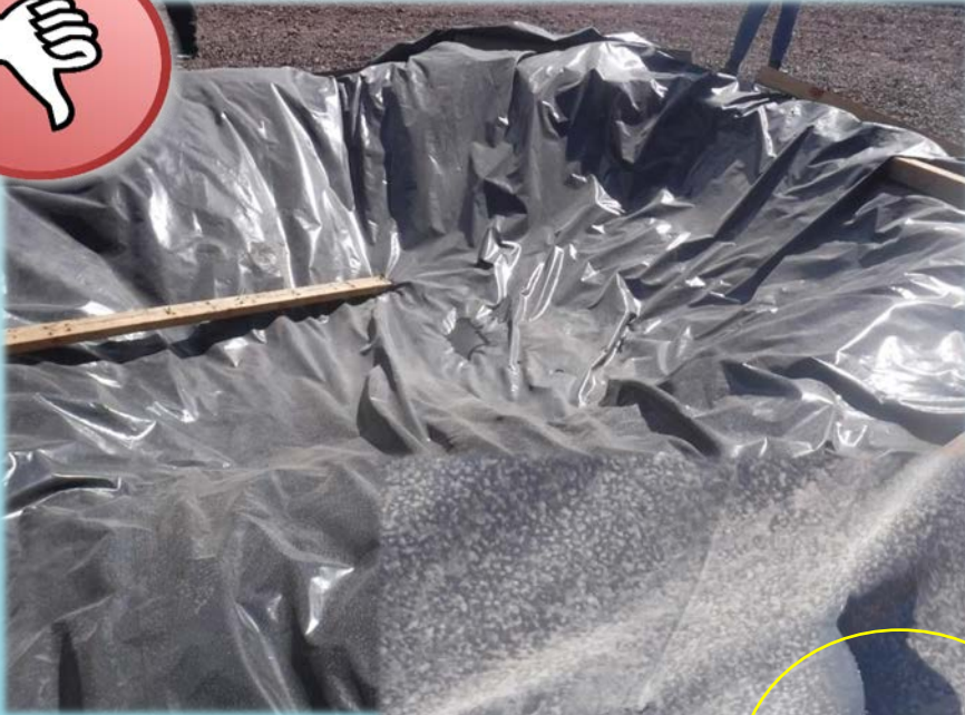
Washout has holes in plastic
