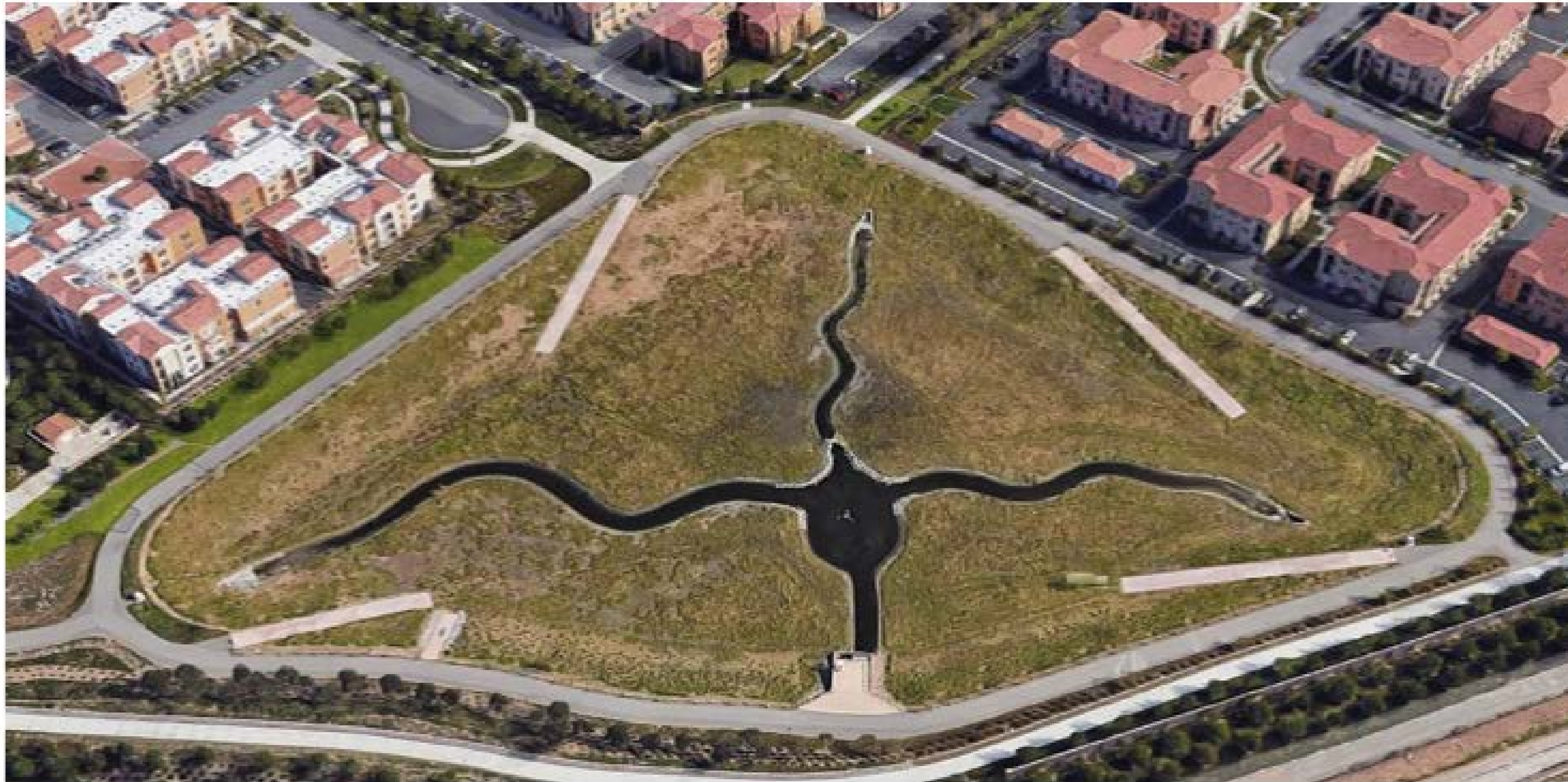
Photograph of a Typical Detention Multi-Benefit Trash Treatment System
