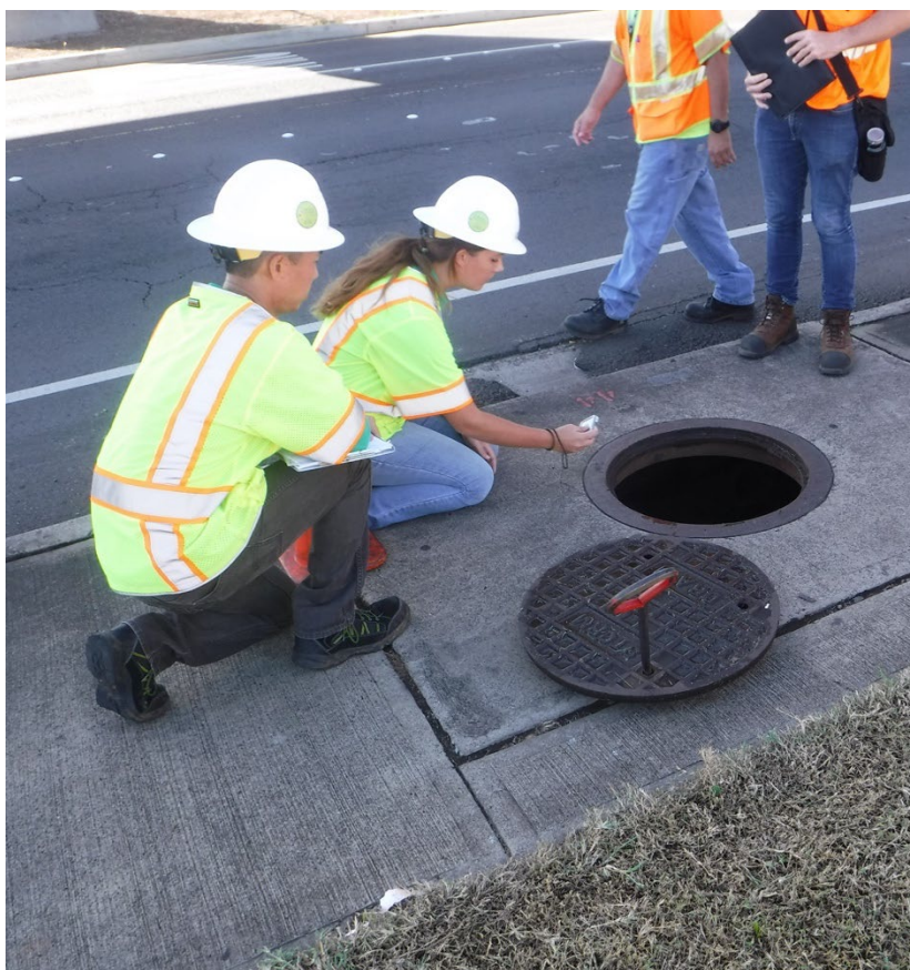
A team of inspectors document a connection.
