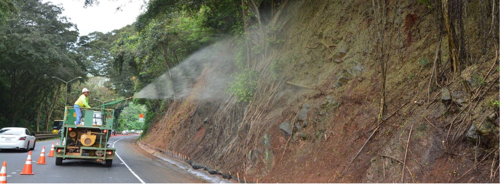
High performance erosion control mulch is used to stabilize significant erosional areas along Kalanianaʻole Highway, Kailua.
