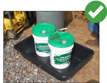
Secondary containment reduces the risk of spills and leaks from getting into storm water runoff, contaminating soil, and injuring workers or visitors.
