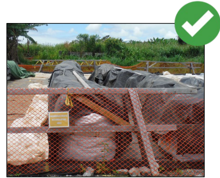
Contaminated material stockpiles must have signage designating material as contaminated.
