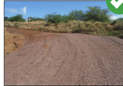
Aggregate used to stabilize temporary construction roads and parking areas must be 2 to 3 inches in size.
