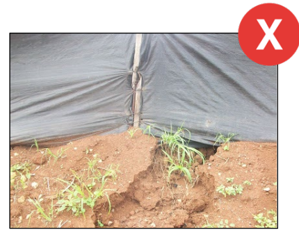
Repair or reinstall silt fence where undercutting has occurred.
