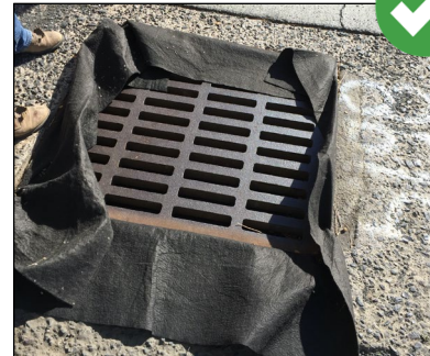
Properly installed geotextile filter fabric is placed underneath the grate and extends 6 inches past the grate on all sides.
