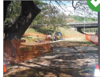
Steel plates were installed under the tree drip line to protect the root system after consultation with a licensed arborist.
