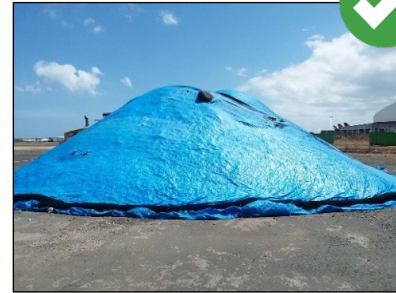
Cover stockpiles with 10 mil plastic sheeting or comparable impermeable material and place perimeter controls 1 to 2 feet from the base of the stockpile.
