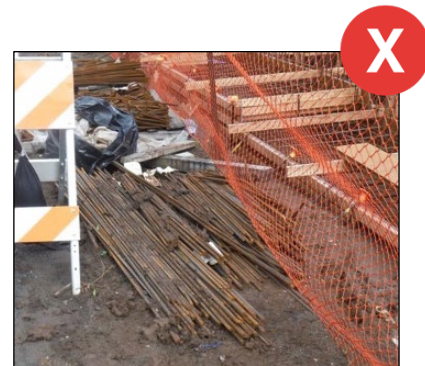
Galvanized metal and rebar must be racked off the ground and covered with impermeable material.
