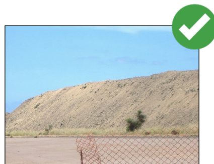
Use a tackifier, netting, or mechanical “punching” method to anchor mulch. Method depends on slope steepness, accessibility, soil conditions, and longevity.
