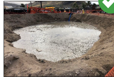
Dewatering pits may be pumped with water from dewatering operations so construction activity may be accomplished.
