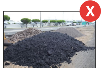
Cold patch spoil piles or waste asphalt piles must be placed on and covered with impervious material, as well as have full perimeter control around the base of the stockpile.
