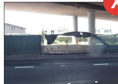
Dust screens must be maintained until permanent ground cover has been established.
