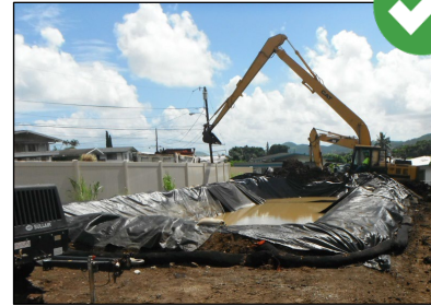
Construct sediment trap prior to engaging in clearing, grubbing, or grading activities.
