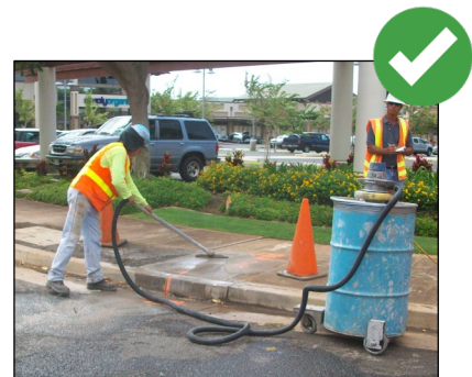
Properly vacuuming saw cut and boring slurry prevents the slurry from entering storm drain systems and adjacent waterbodies.
