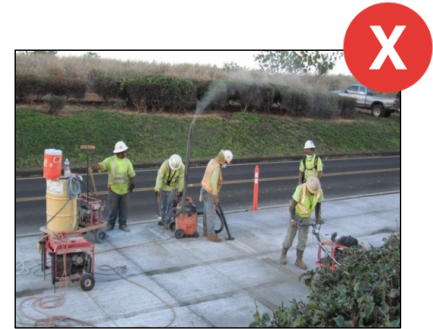
Vacuuming without a filter creates a dust cloud of sawcutting fines.
