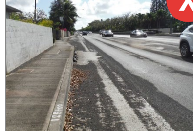
Asphalt waste and debris must not enter storm drainage systems or waterbodies.
