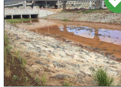
Inlets, outlets, and slopes of sediment basins must be stabilized with rock or vegetation to minimize erosion.
