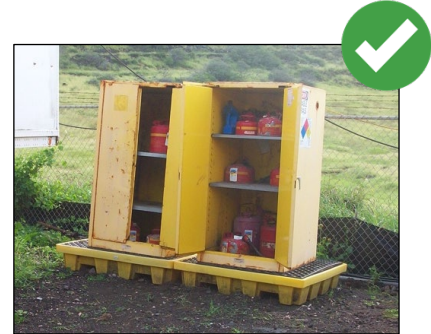
Hazardous materials stored under a covered facility and in secondary containment prevents storm water from coming into contact with materials.
