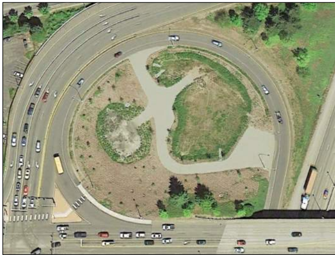
SOURCE: Google Earth (I-5 Exit 102, Tumwater, Washington)
