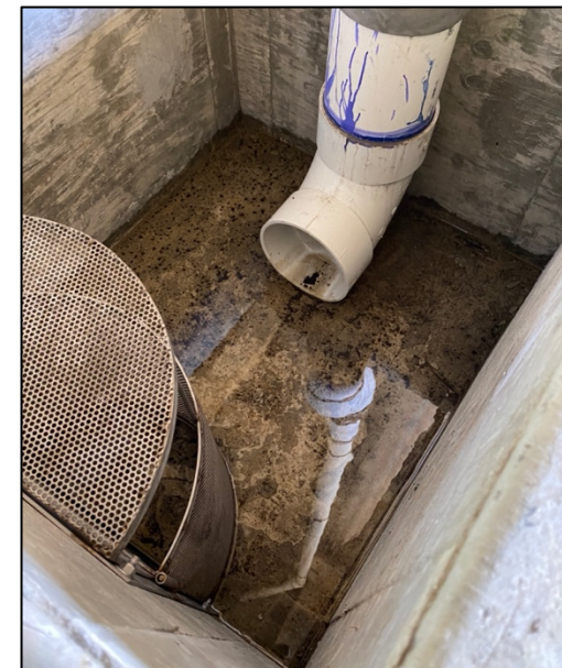
Newly Constructed Downspout Filter Box
