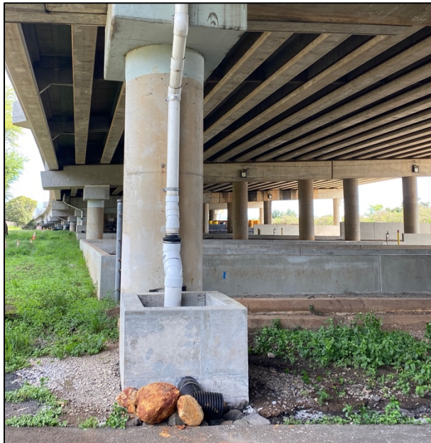
Newly Constructed Downspout Filter Box
