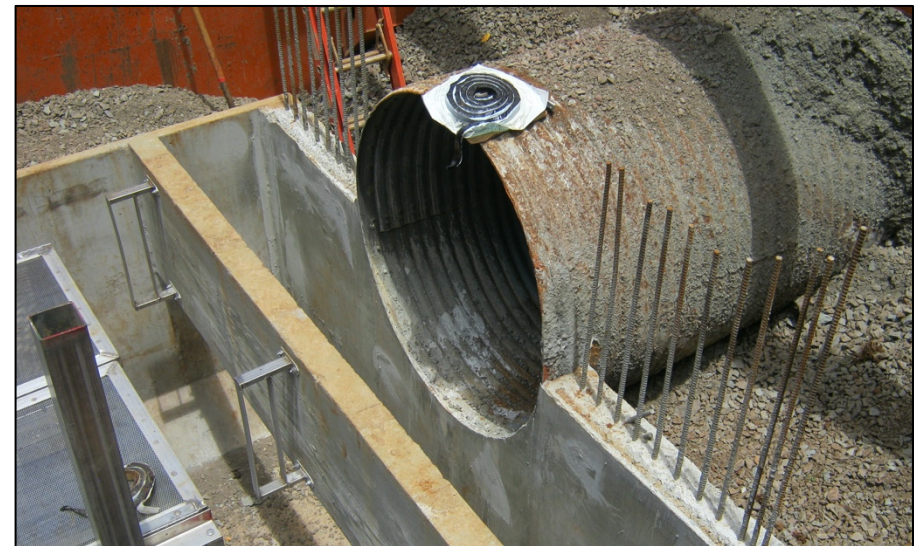
Nutrient Separating Baffle Box during construction
