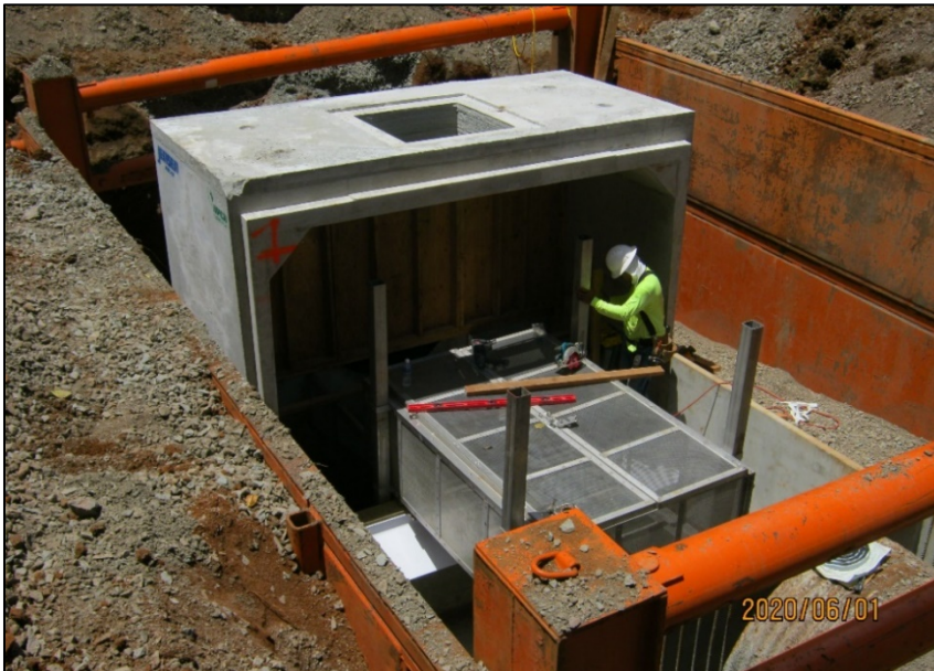
Nutrient Separating Baffle Box during Construction
