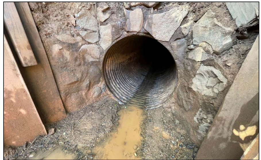
Outfall after removing debris
