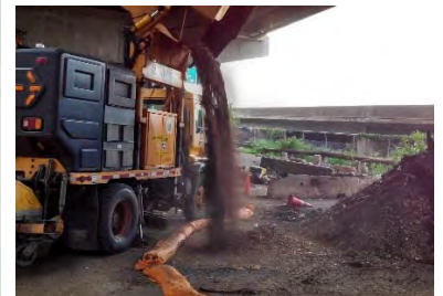
Use berms for stockpiling.
