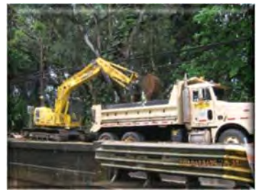
Remove material from work site.
