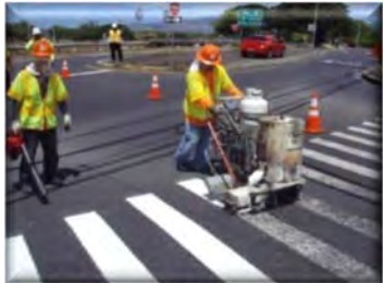
Protect storm drains.
