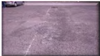
Clean up work site.
