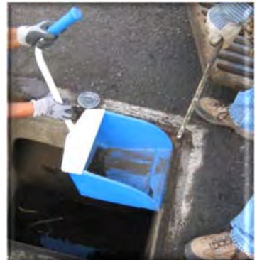
Clean storm drain.
