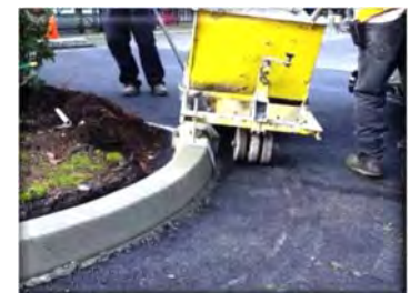
Repairing a curb.
