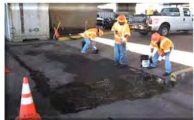
Complete repair work.
