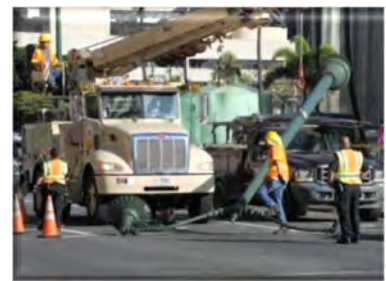
Collect debris safely.
