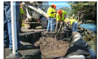
Protect surface water.
