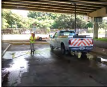
Wash vehicles within containment.
