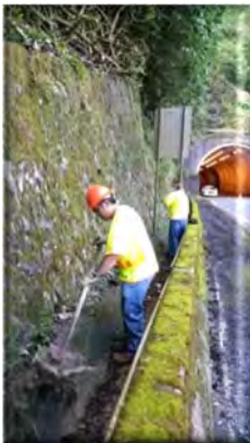
Shovel dirt and debris.
