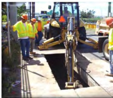
Expose the buried utility.
