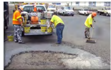
Clean up debris.
