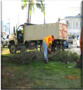
Remove and dispose of debris.
