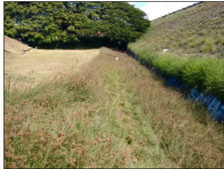
H-1 Freeway Eastbound Onramp Cloverleaf, Mo'ili'i, Hawaii
