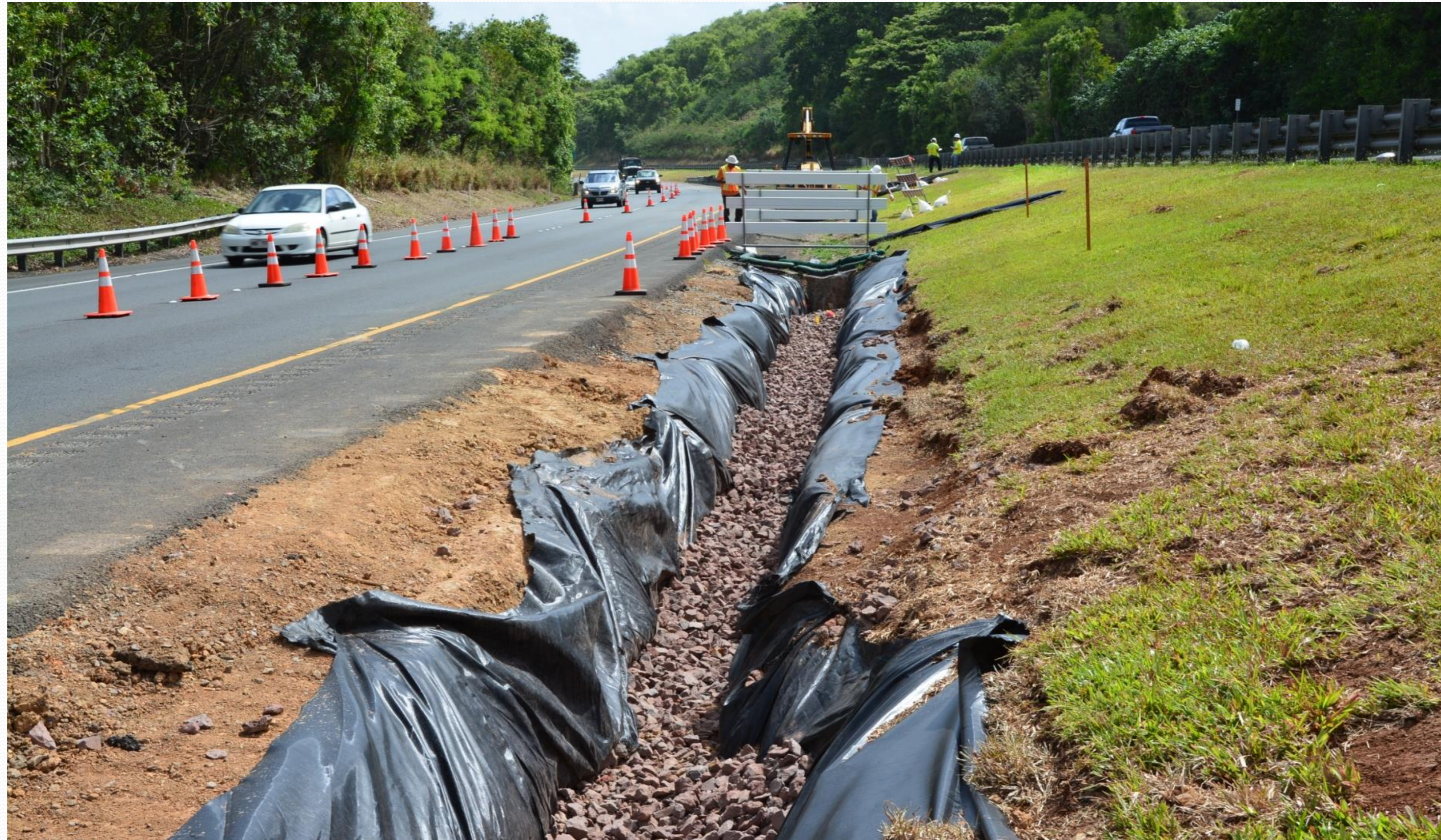
Enhanced/Bioswale Construction
