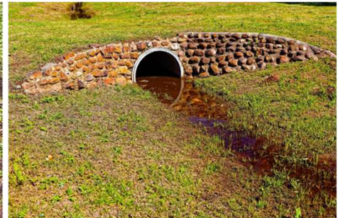
Right examples of rip rap around outfalls to prevent erosion.
